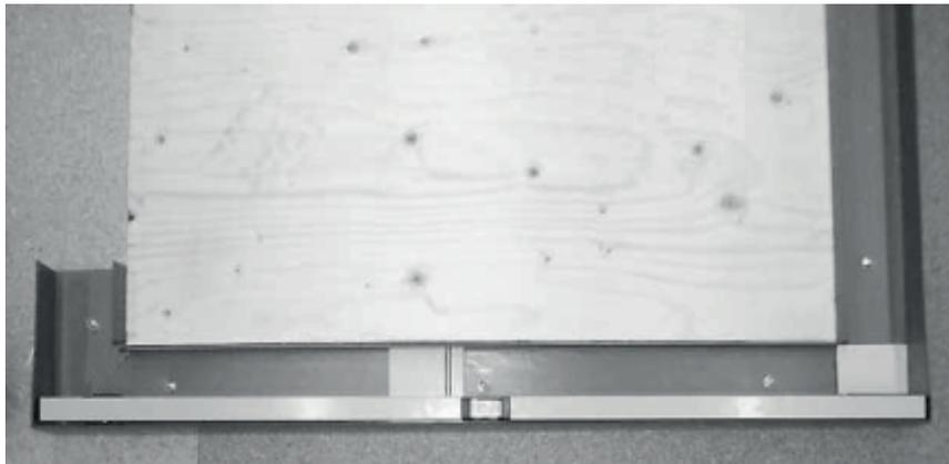
It is recommended that there should be no more than 3mm tolerance in the floor level, as this can affect the correct location of the panels.
