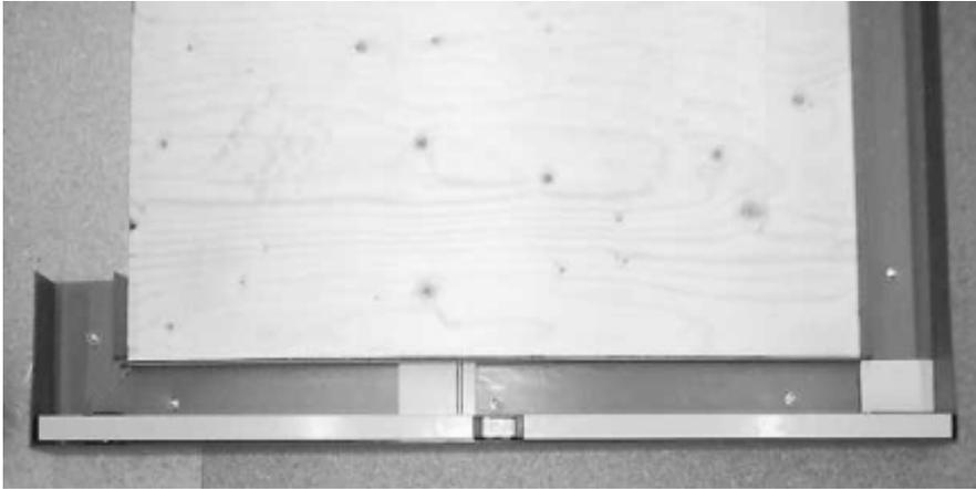
It is recommended that there should be no more than 3mm tolerance in the floor level as this can affect the correct location of the locking panels.
